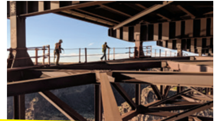
EXTREMES WJE teams assess the Chicago Skyway Bridge (above left) and a 1,500-ft-long deck truss-arch of the Perrine Bridge over the Snake River in Idaho.
