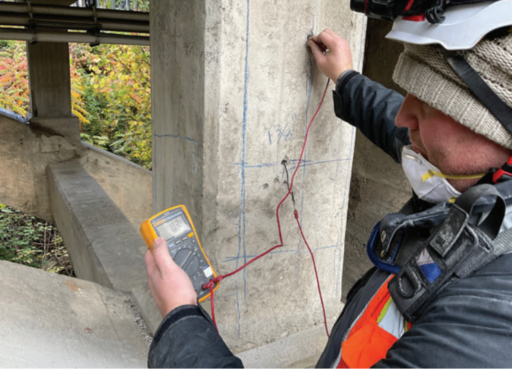
Fig. 4: Rebar continuity verification
