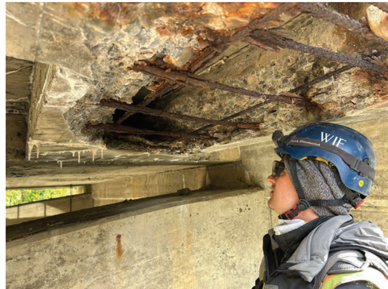
Fig. 3a: Example of corrosion in reinforced concrete; corrosion and spalling near drain
