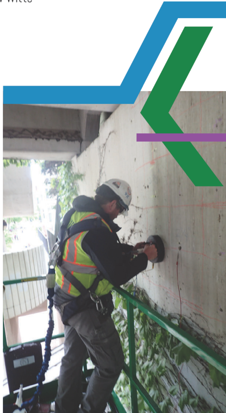
Corrosion rate testing of reinforced concrete
