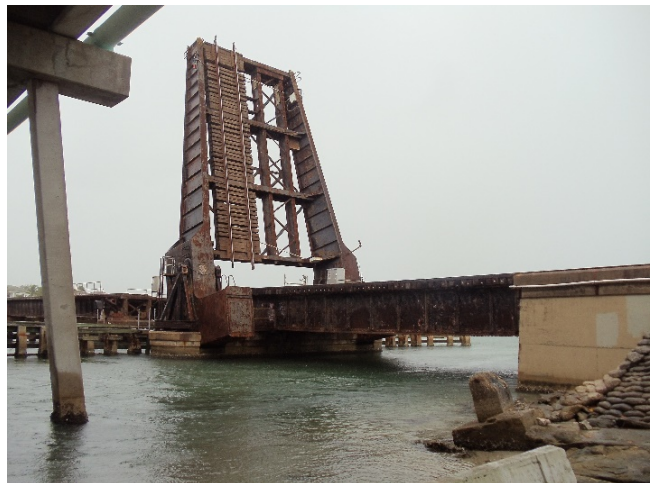
Existing Bascule Span in the Raised Position
