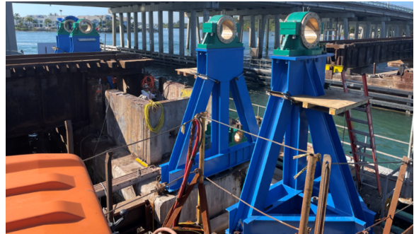
Towers installed and aligned on pier
