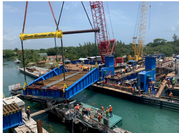
Lifting toe section into place
