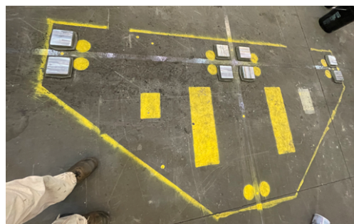
Layout of sole plates to support towers at shop assembly
