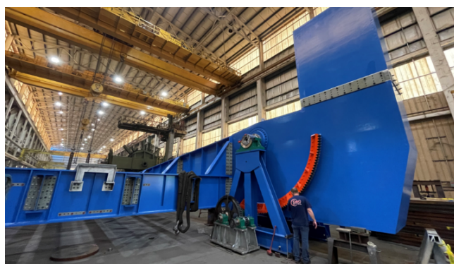
Completed shop assembly of leaf supported on towers
