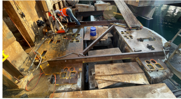
Tower template installed on bascule pier
