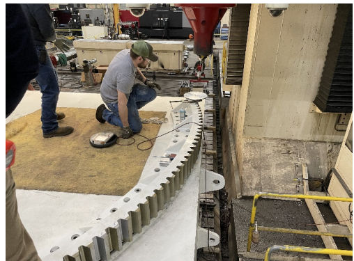
Checking rack alignment on the mill
