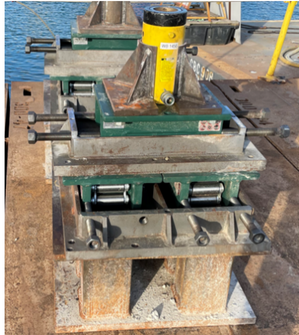
Manipulator to aid alignment of toe section
