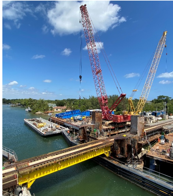
Flying jump span installed and open for train traffic
