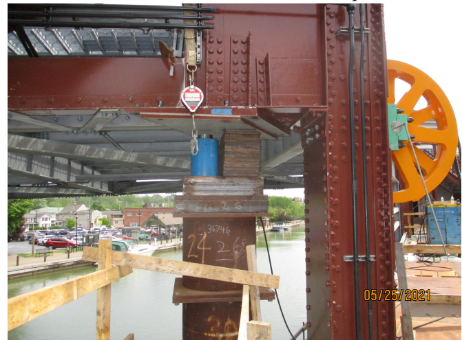
Figure 4 –Jacking Column for Span Support
