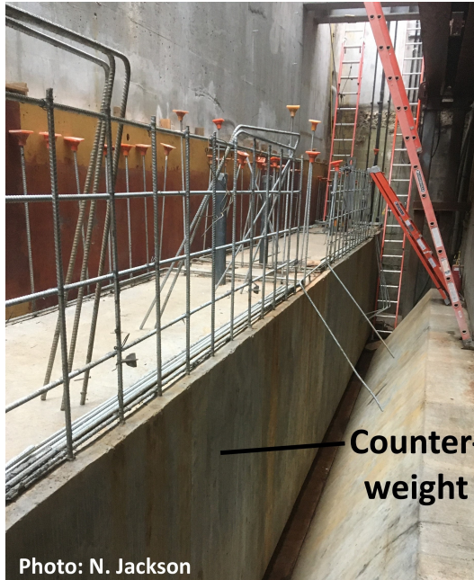
Figure 5 –New Counterweight at Interim Stage of Construction
