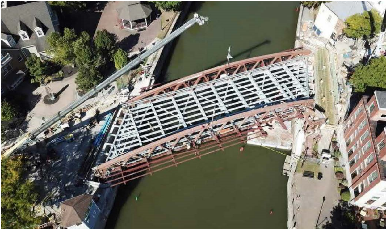
Figure 3 – Aerial View of framing during rehabilitation illustrating skew geometry.
