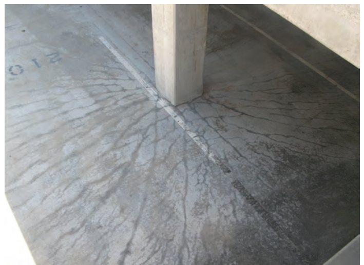
Fig. 1. Radial cracking appears in the two-way floor slabs of a garage built circa 1985 (left) and a garage built circa 2008 (right). Both structures are still in service.
