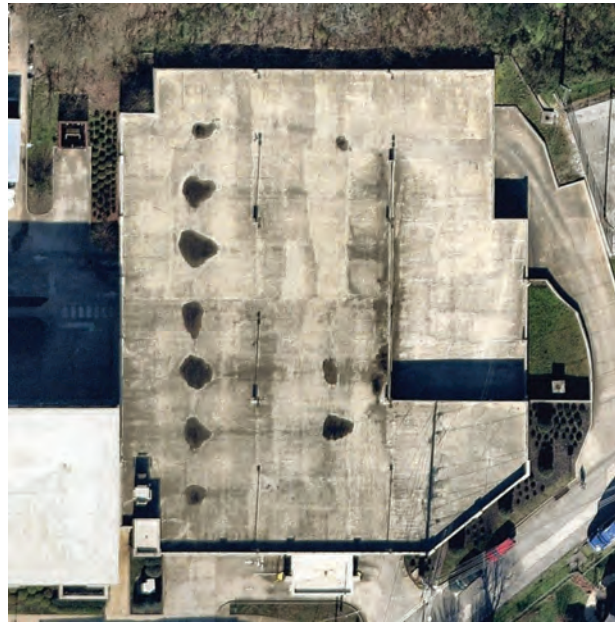
Fig. 3. Mid-bay puddles in a parking structure roof slab are due to the unavoidable deflection of the roof slab between columns. Photo courtesy of www.nearmap.com .
