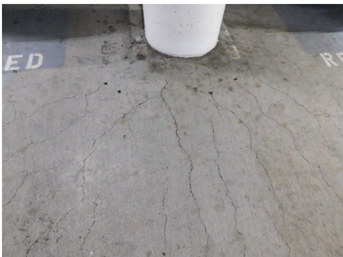
Fig. 1. Radial cracking appears in the two-way floor slabs of a garage built circa 1985 (left) and a garage built circa 2008 (right). Both structures are still in service.
