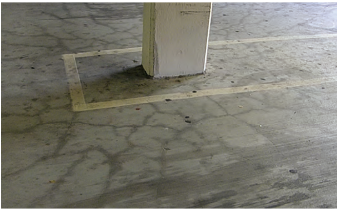
Fig. 2. Spiderweb cracking appears in the two-way slabs of a garage built circa 1991 (left) and a garage built circa 1987 (right). Both structures continue to function without issue more than three decades after they were built.
