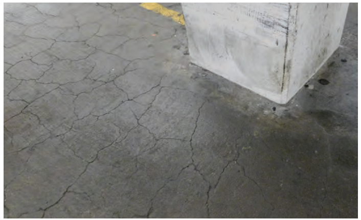
Fig. 2. Spiderweb cracking appears in the two-way slabs of a garage built circa 1991 (left) and a garage built circa 1987 (right). Both structures continue to function without issue more than three decades after they were built.
