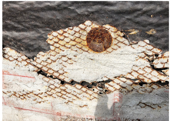
Figure 2. Corroded Lath
