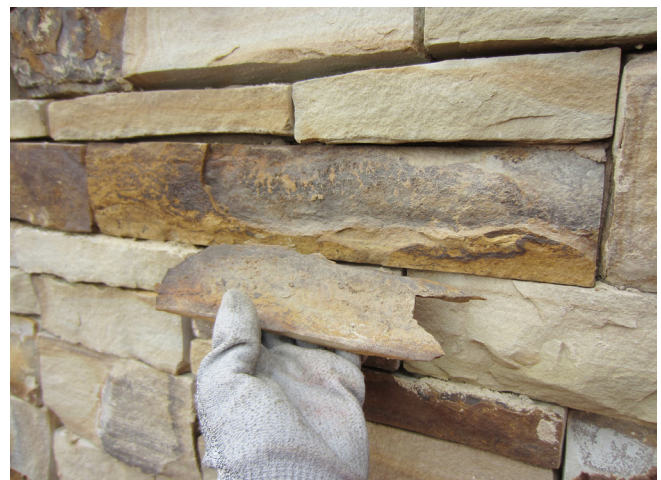
Figure 3. Delaminated Stone
