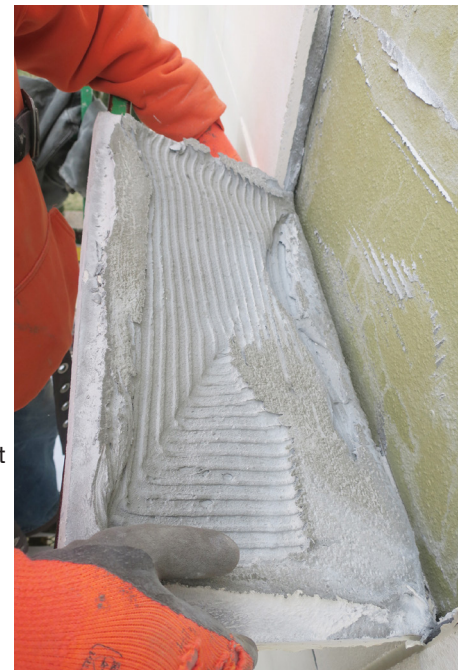
Figure 4. Limited Adhesive Coverage
